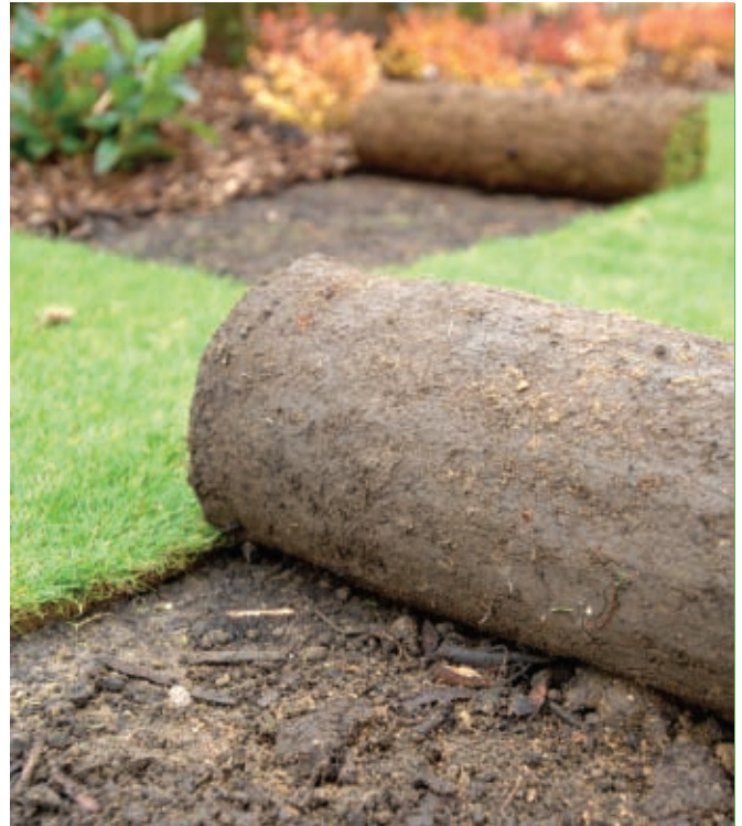
Turf laid onto manufactured topsoil at Countryside Properties development, Hampton Vale, Peterborough.
